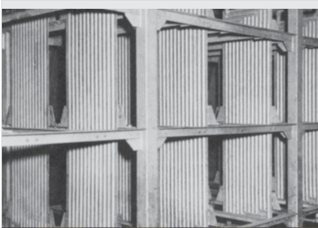
Built-in aqueduct for cooling engine jacket water
