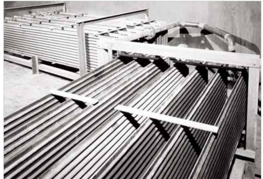
PLATECOIL banks for heating viscous products in large petroleum storage tank
