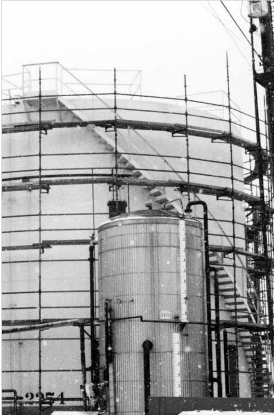
Clamp-on PLATECOIL for a large storage tank
