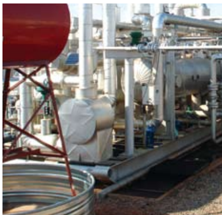
Compact, skid-mounted propane condenser.
